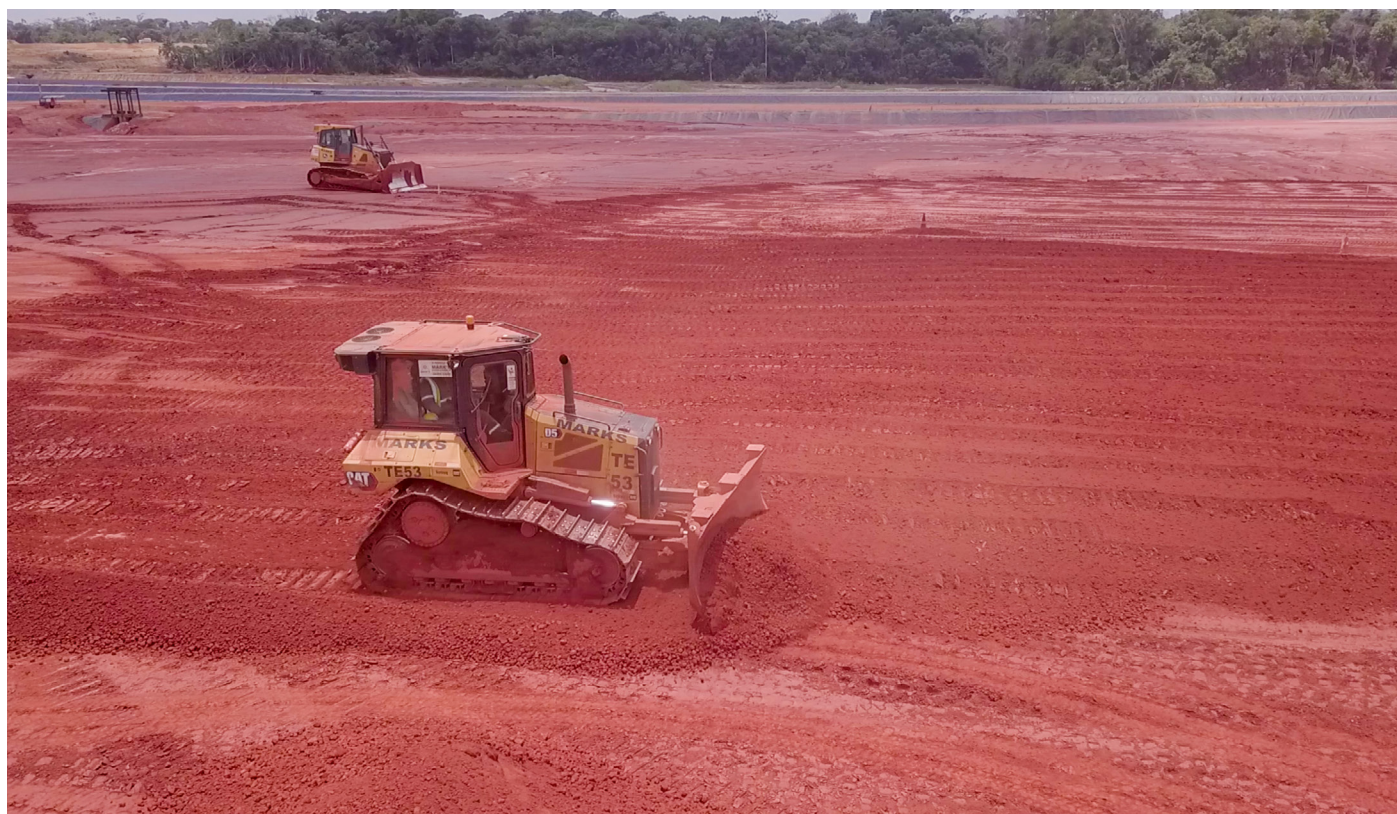
Figure 16. Dry Stacking Residue from Press Filters
